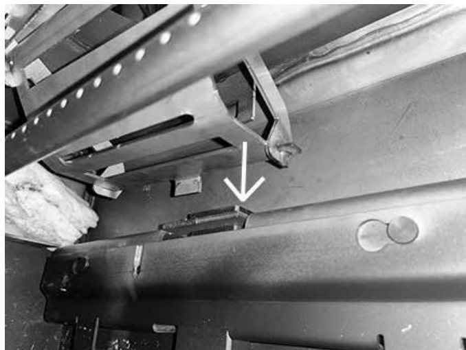
Figure 3: Remove Flue Gas Agitator
