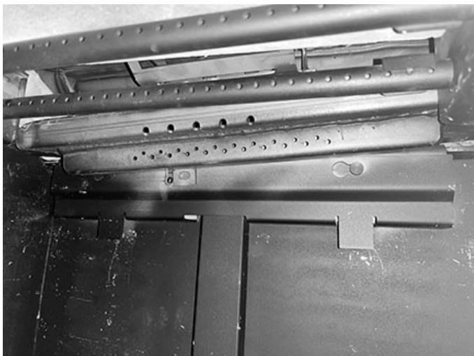
Figure 2: Remove rear baffle.
