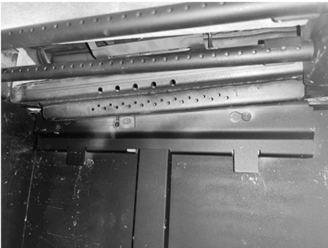
Figure 4: Remove rear baffle.
