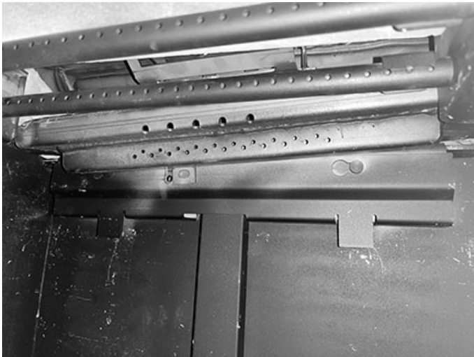
Figure 7: Remove rear baffle.
