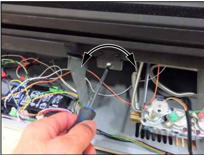
Figure 59: Primary Air Adjustment
