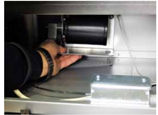
Figure 64: Placing Left Fan in Place
