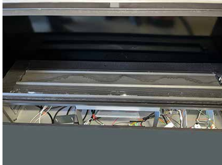
Figure 67: Burner panel Removal
