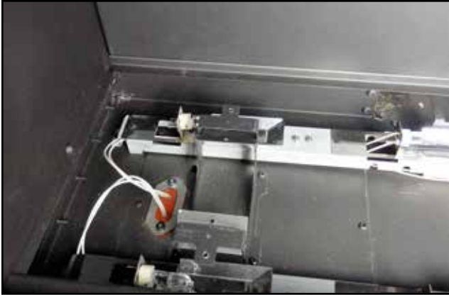
Figure 87: Ember Lights Wiring Installed
