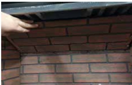
Figure 69: Top Panel Install B.
