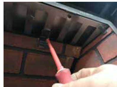
Figure 70: Top Panel Clips.
