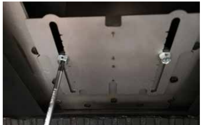
Figure 88: Sliding Damper.
