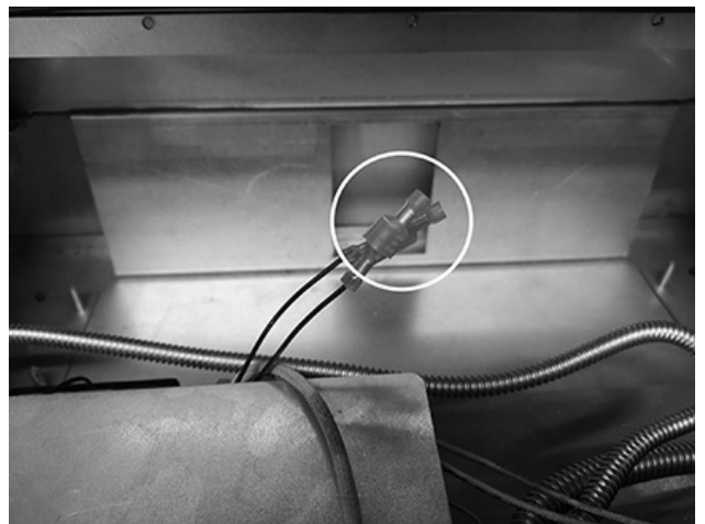
Figure 63: Remove the male connectors.
