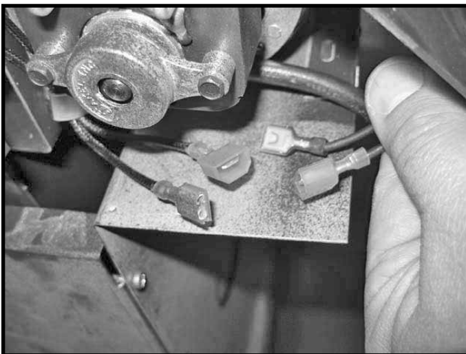
Figure 21: Disconnecting fan wires.
