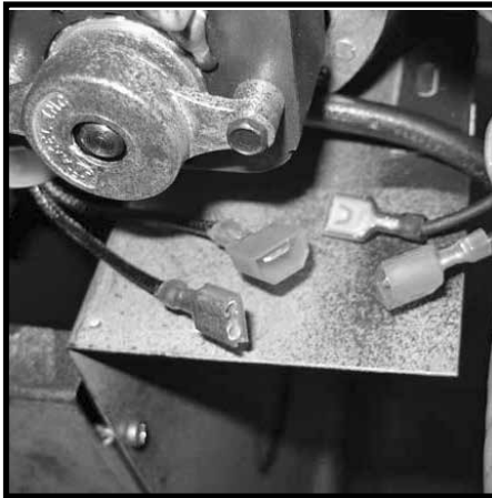
Figure 13: Disconnecting fan wires.
