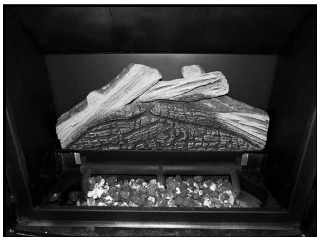
Figure 46: Number 1 log set in place.
